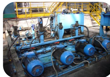
Piping and mounting
