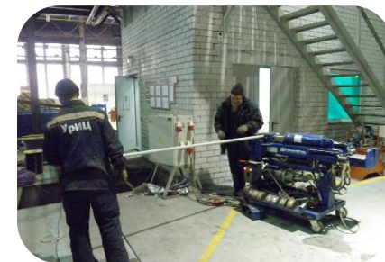
Piping and mounting
