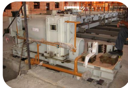
presses and forging complexes
