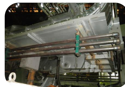
Mounting and flushing of pipelines
