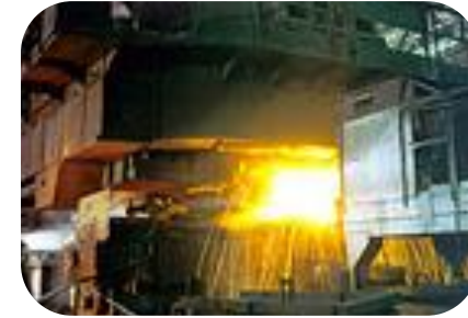
Continuous steel casting machines
