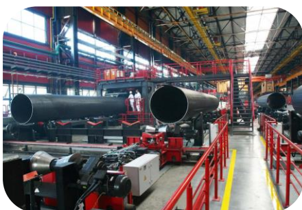
Complex reconstruction of pipe rolling
