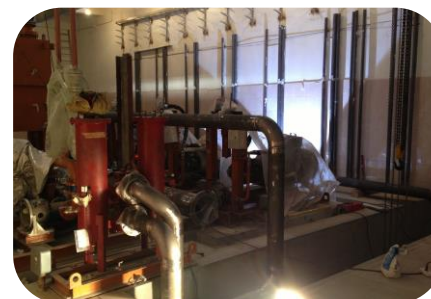
Etching, flushing and pressure molding of pipelines of lubrication systems
