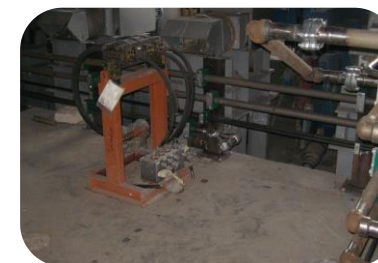
Installation and flushing of pipelines
